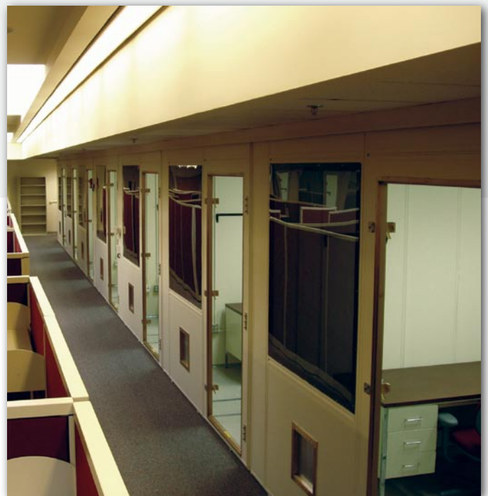
Complex consisting of nine shielded anechoic enclosures. Installed at DNB Engineering, Inc. Fullerton, CA.
