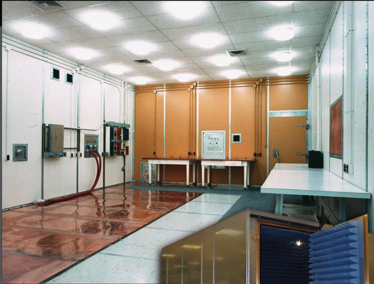
USC Turnkey Installation
